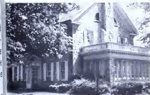
Penn Mutual Insurance Company building at 2921 North Front Street; Pocono sandstone.
